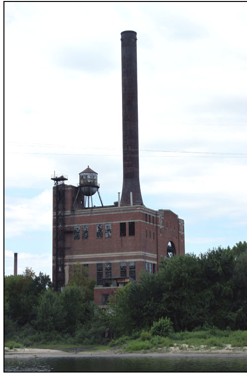
Figure 20. Island Station, looking northwest, 8/17/12. (Christine Boulware)
