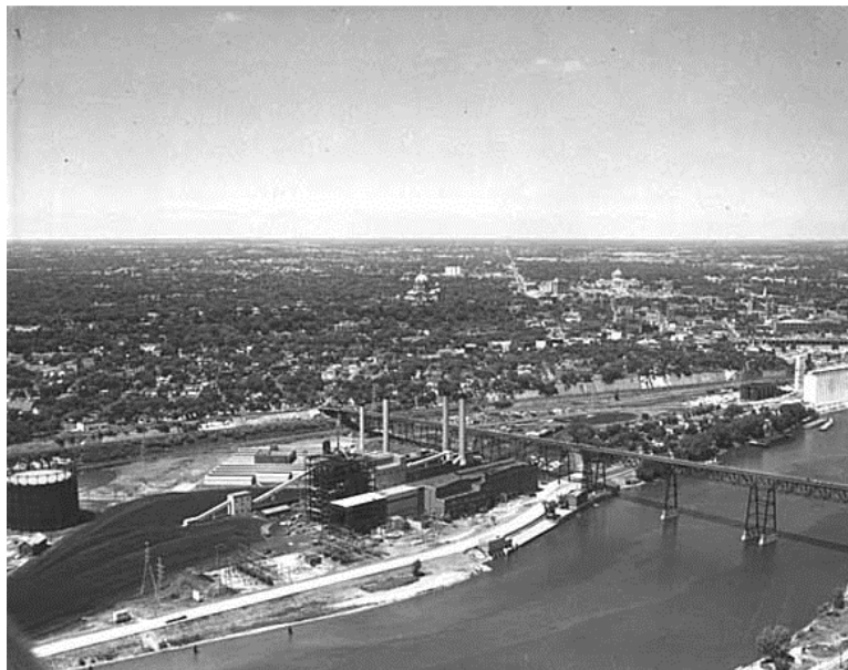
Figure 14. NSP High Bridge Plant (1924), in 1958, looking northeast.
