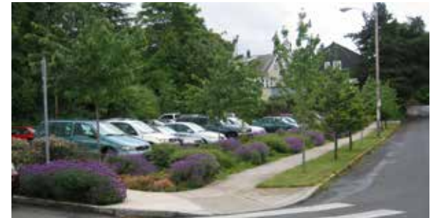
Landscaped parking lot edging with stormwater management areas.
