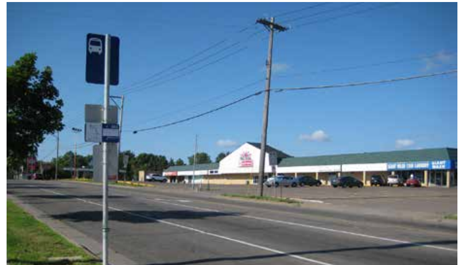
Photo of catalyst site #2 (Short-term redevelopment recommendation)
