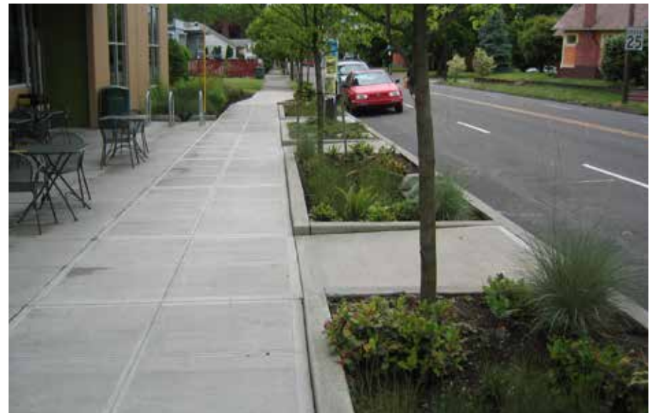
Examples of infiltration and flow-through planters
