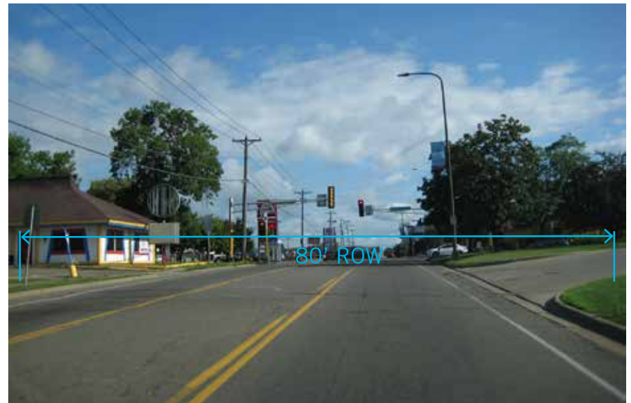
Photo of existing Rice Street 80' ROW (south of Larpenteur Avenue)
