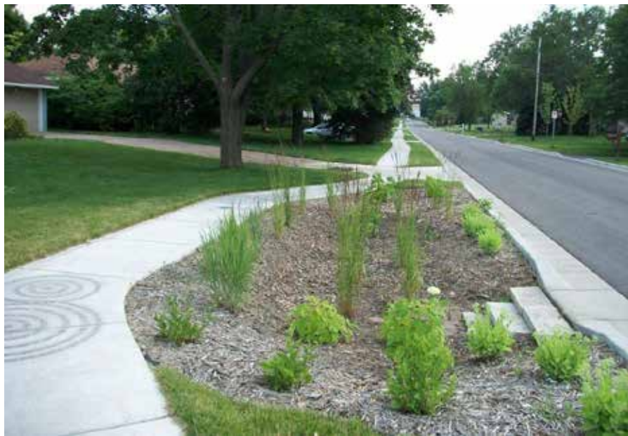
Example of vegetated swale in Maplewood
