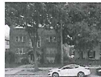
GRAND AVE STREET VIEW
