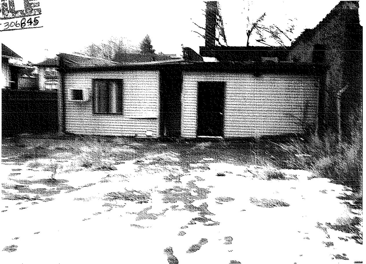
Back of ex building (to be removed)
