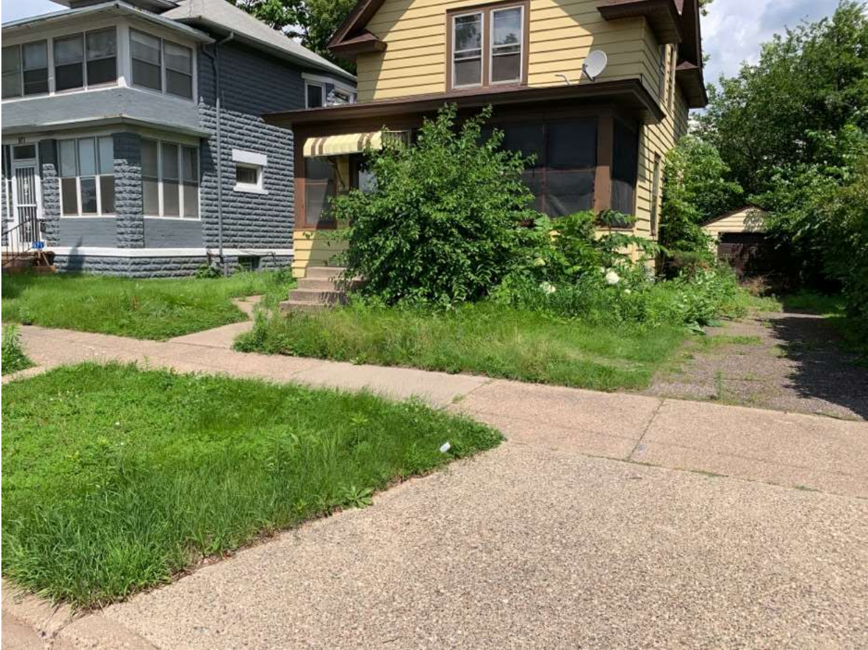
967 St Anthony Ave.Recheck on 7/9/24 - Photos
