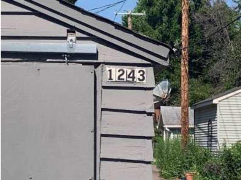
1243 Thomas Ave rechecked photos 7-16-24
