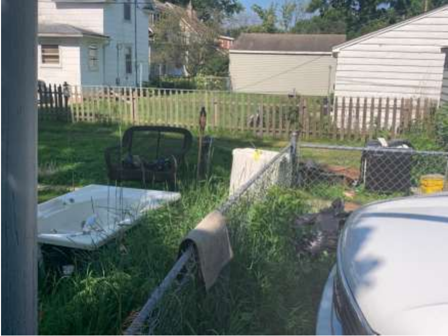
1243 Thomas Ave rechecked photos 7-16-24
