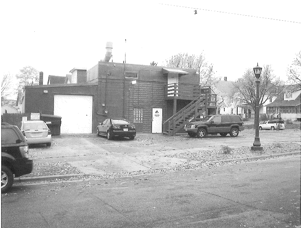
Subject site as viewed from Maple Street
