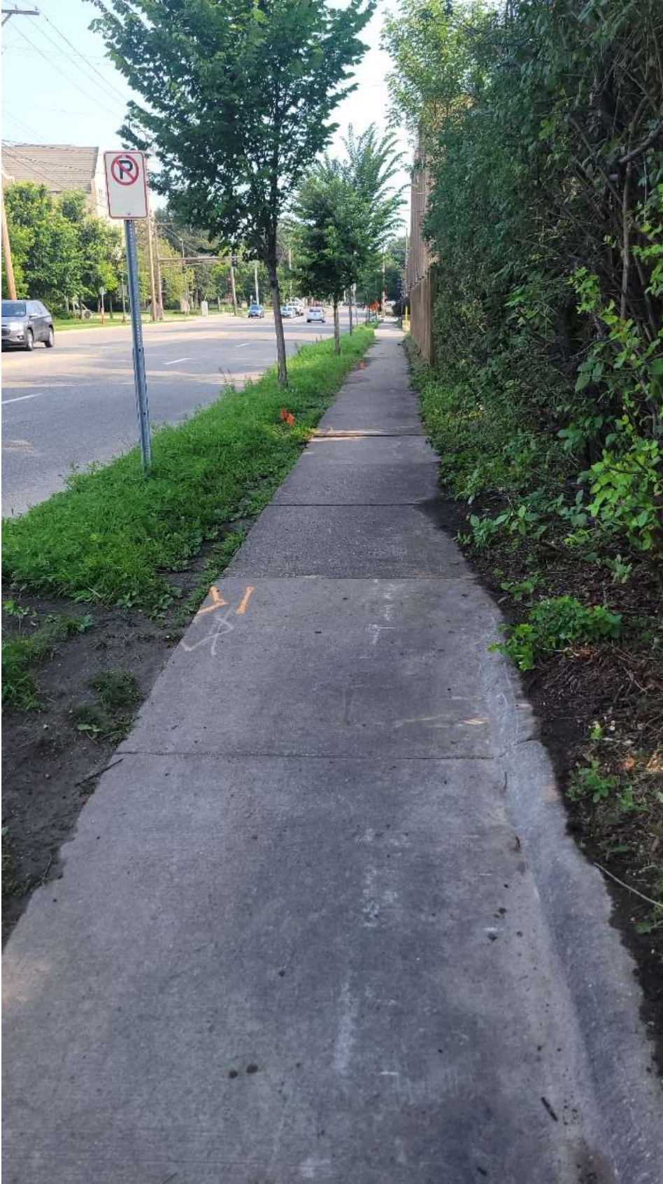
Contractor work done 7/22/24 (loaded to system 8/2/24)
