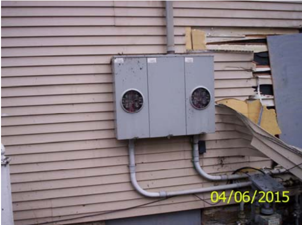
Electric meters pulled
