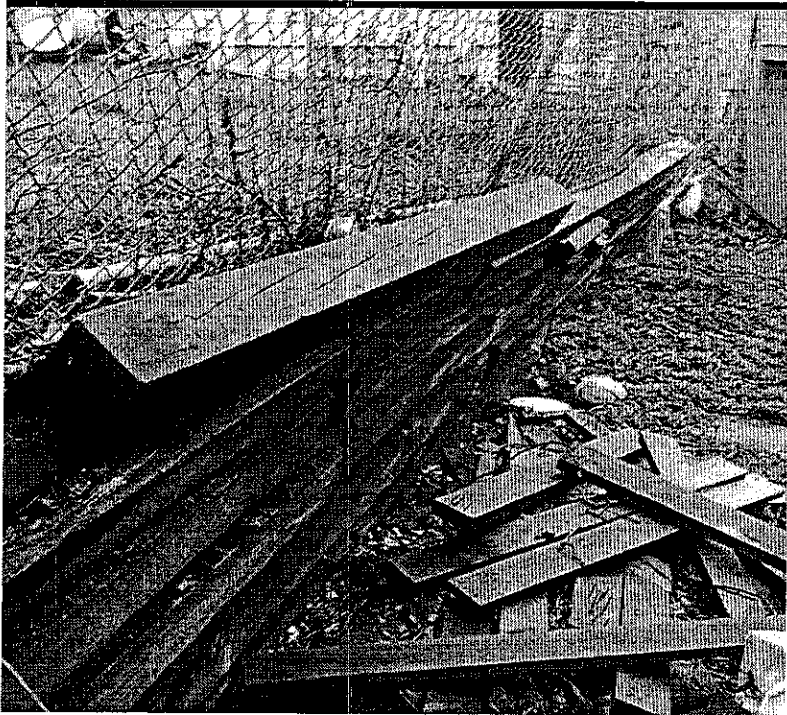
This is the middle of our properties the 2 x 4 nailed to the wall is where the neighbors use to climb
