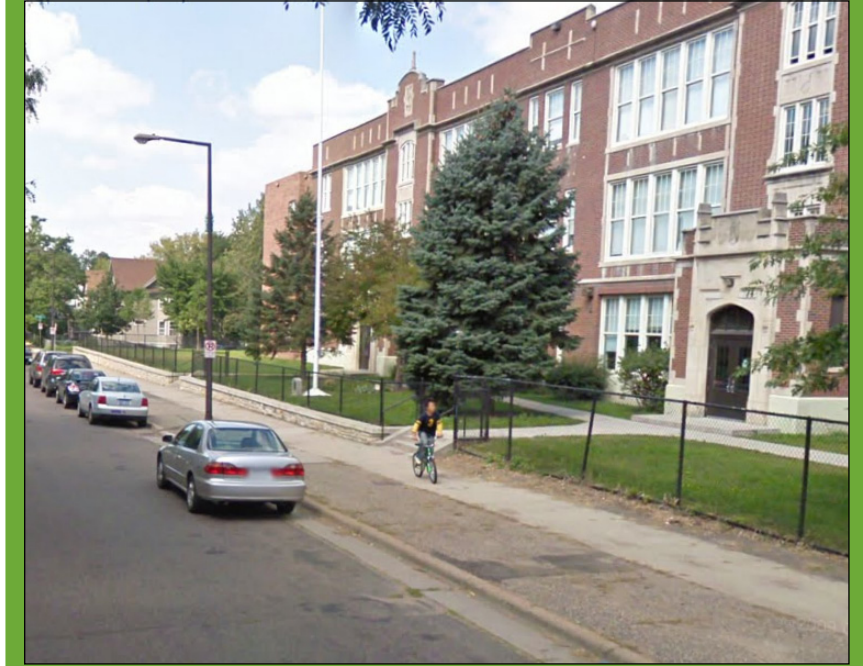
FIGURE 3.6 - A series of targeted streetscape improvements around Jackson Elementary School will help to make it safer and more comfortable for people to walk to and from the school.
