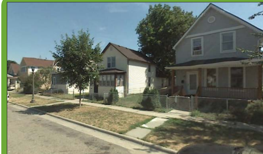
FIGURE 1.7 - North of University Avenue, the area is comprised of blocks of early 20th century housing served by rear alleys. In recent years, this area has been severely hit by foreclosures and vacancies.
