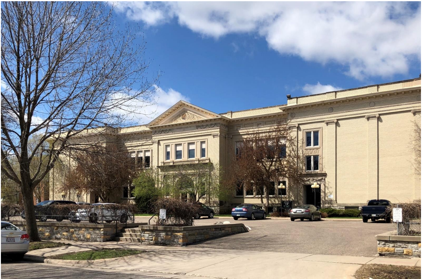
Professional office building at 1619 Dayton Avenue - looking north
