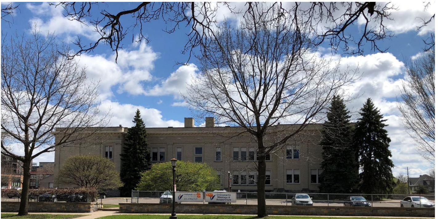
Site of proposed apartment building along Marshall Avenue - looking south
