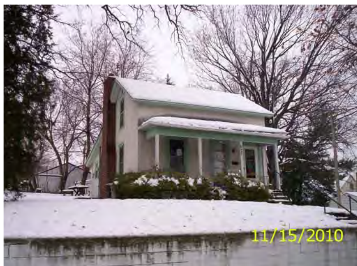
South and east sides, posting
