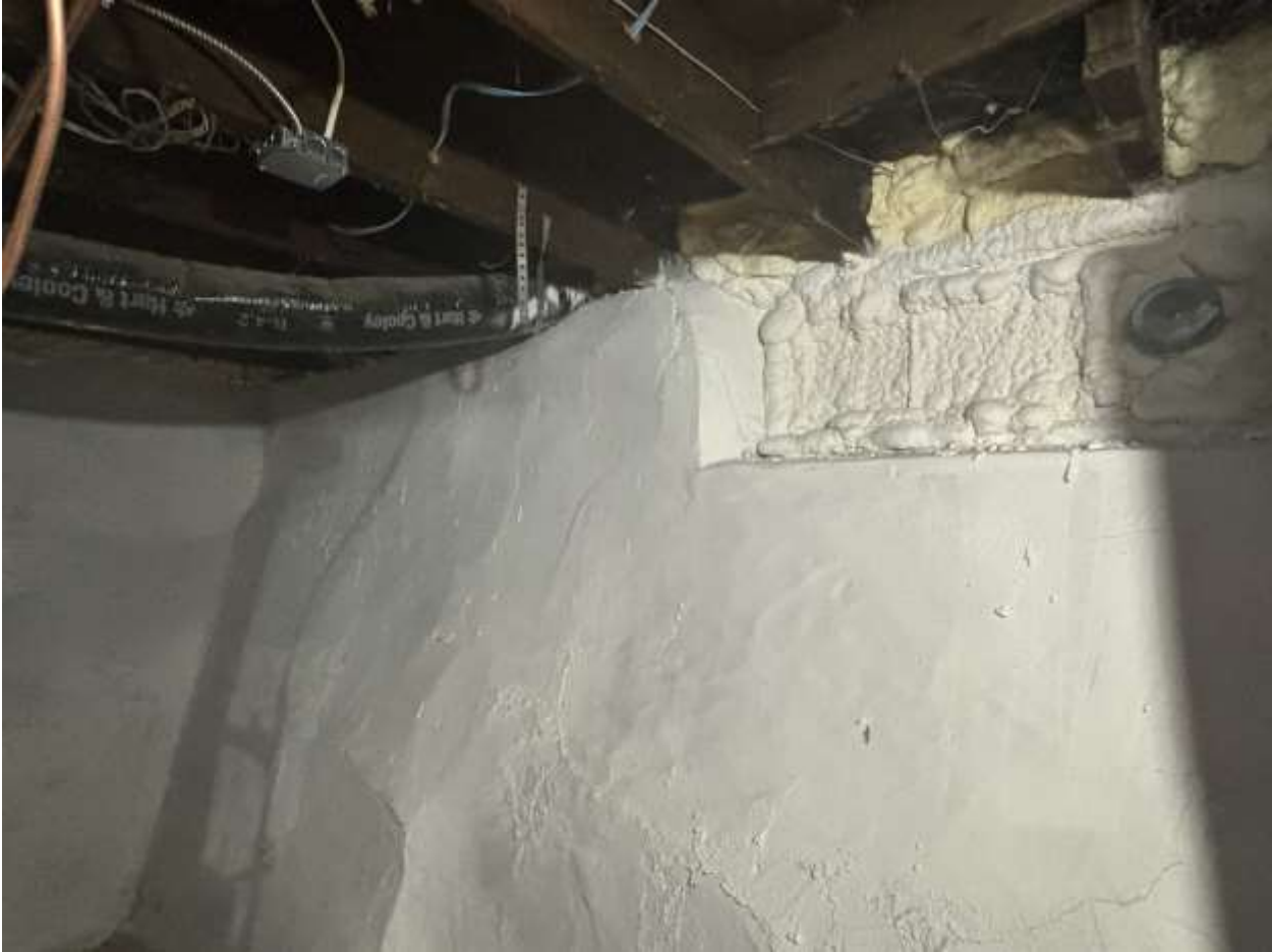
705 Magnolia Ave screen dryer vent
