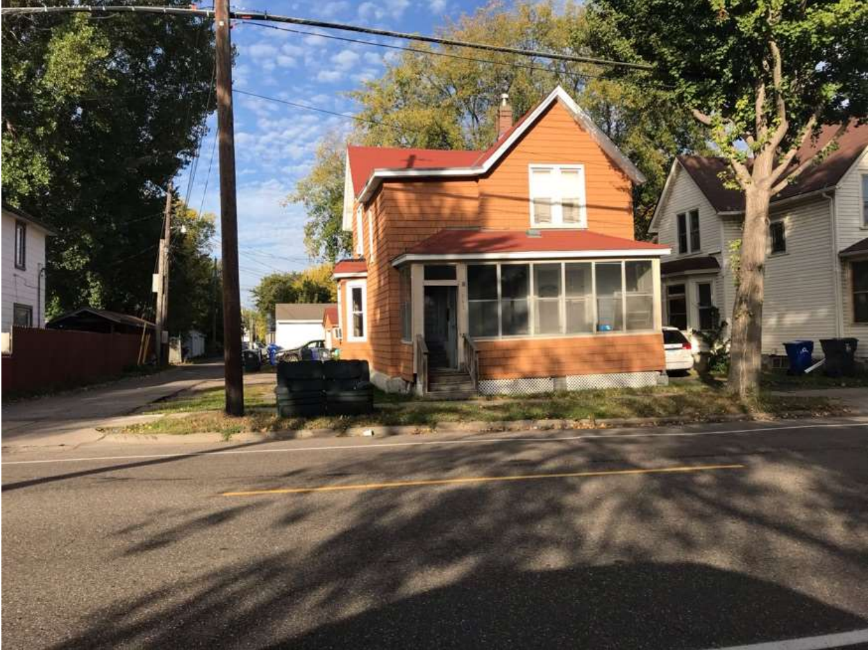
649 Western Ave N.Photos.10-6-20 rechecked
