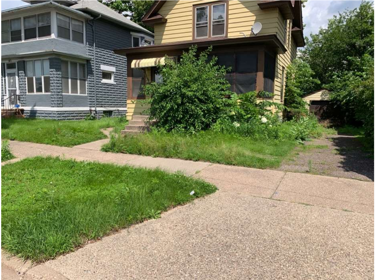
967 St Anthony Ave.Recheck on 7/9/24 - Photos
