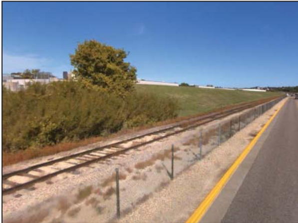
View of Levee from Airport Road
