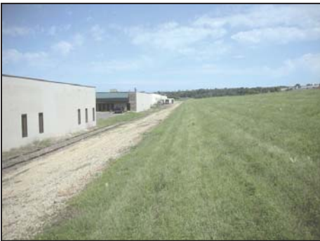
Back side of Levee near Holman Field.
