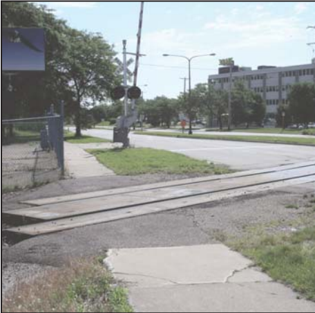
Track Crossing Plato Blvd. & Starky St.
