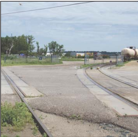
Track Crossings at Barge Channel Rd.
