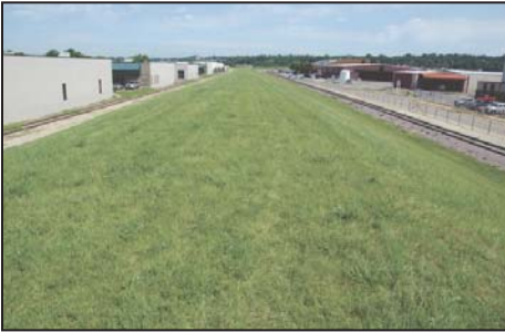
Top of levee along Airport Rd.
