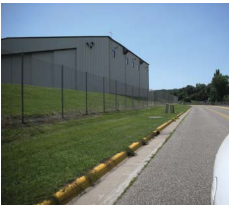
Airport Rd. showing proposed trail location
