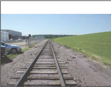
Tracks adjacent to levee at Airport Rd.
