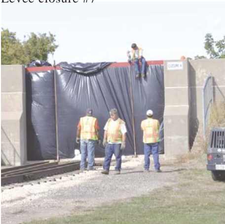
Preparing levee closure for flood conditions
