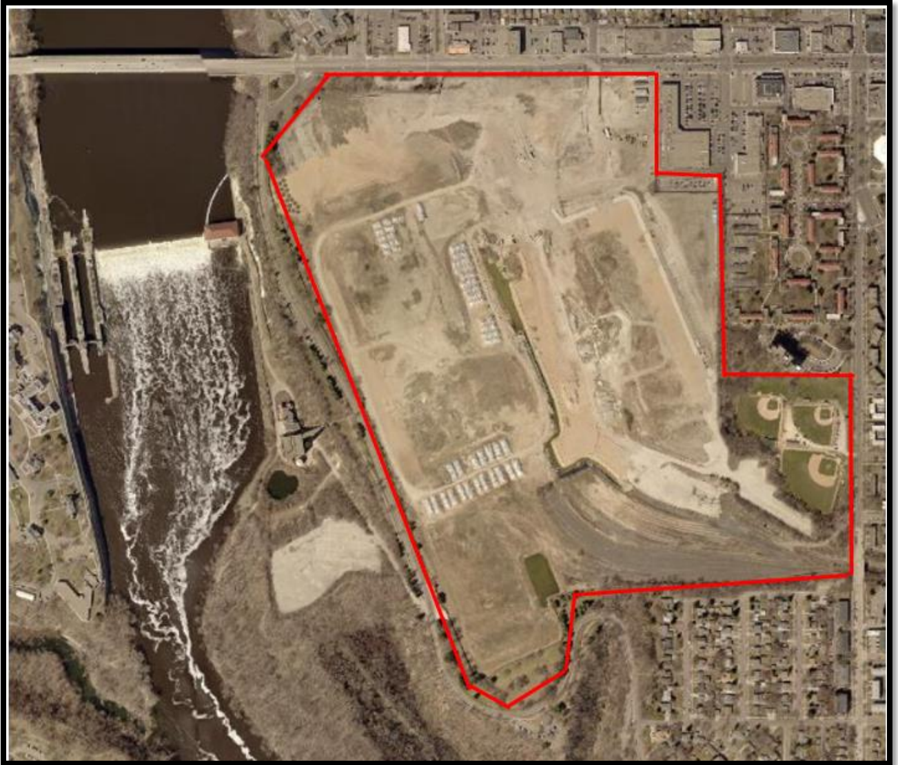
Photograph provided by Ramsey County GIS.
