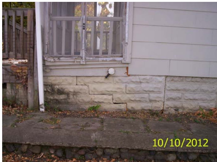
Deteriorated blocks
