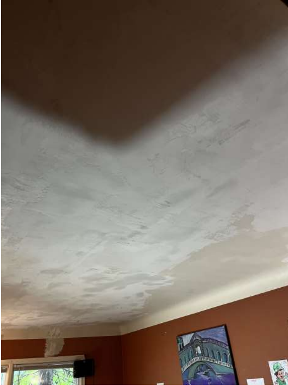
1220 Sherburne Ave. repair photos by Valmyr 5-20-25
