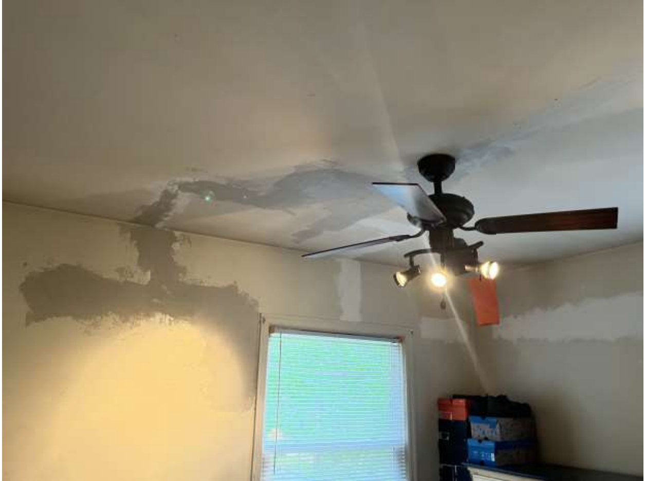
1220 Sherburne Ave. repair photos by Valmyr 5-20-25
