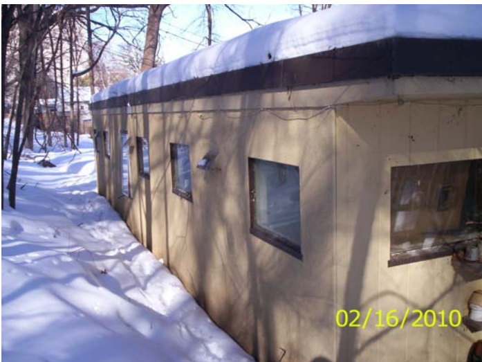
West side house
