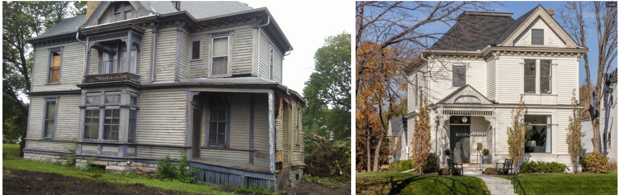
1899 Iglehart, The A.F. Gauger House, 'Before' and 'After' renovation
