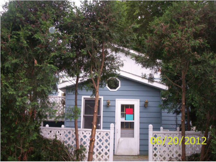
North side, posting
