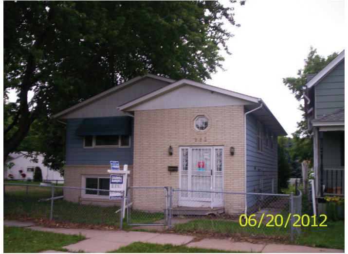
South and east sides, posting
