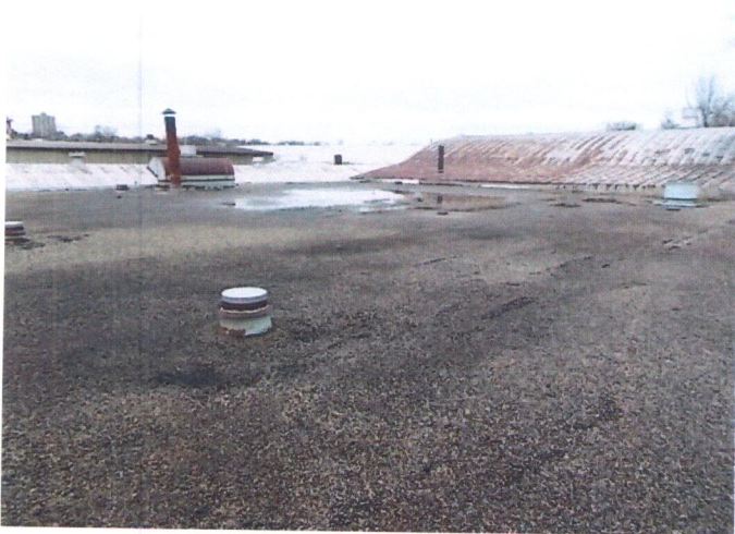
Overall view of roof
