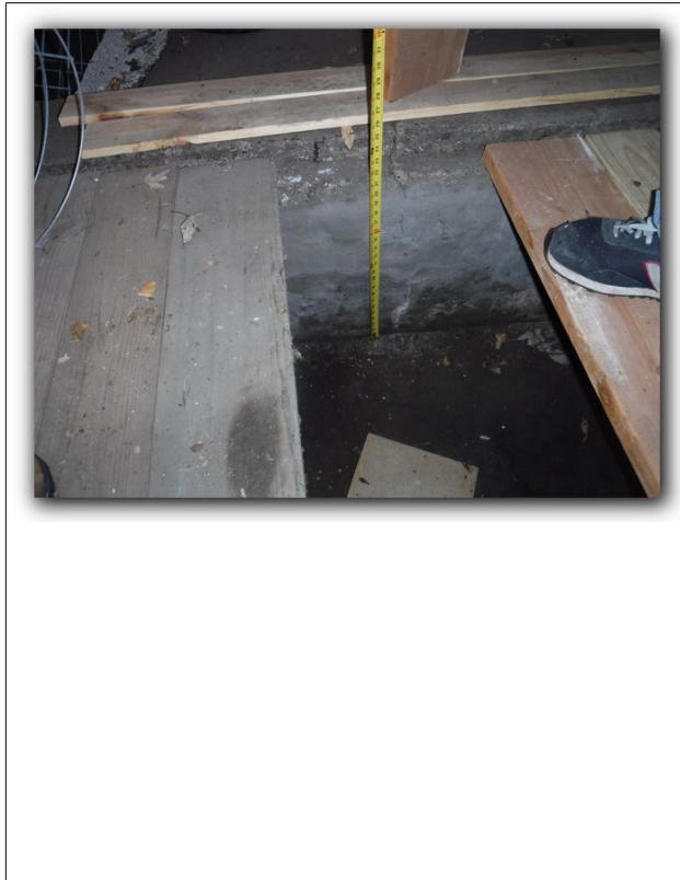
11 "Work trench" at garage floor. Fill with compacted sand and top with concrete.
