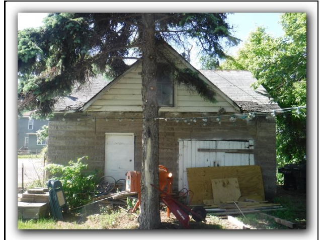
2 West side of garage.
