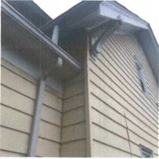
Exterior Walls (Siding/ Stucco/ Brick) (1/3) 08/28/2020 12:26 PM
