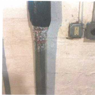
Dryer Vent (3/6) 08/28/2020 12:22 PM
