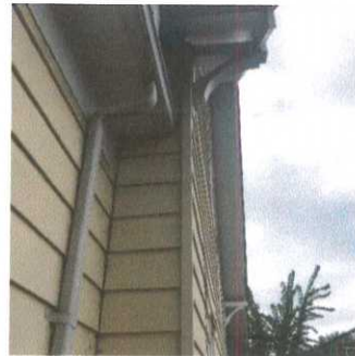
Exterior Walls (Siding/ Stucco/ Brick) (3/3) 08/28/2020 12:26 PM
