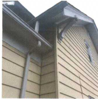
Exterior Walls (Siding/ Stucco/ Brick) (2/3) 08/28/2020 12:26 PM
