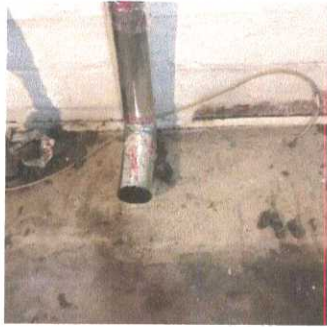
Dryer Vent (2/6) 08/28/2020 12:22 PM
