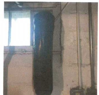
Dryer Vent (4/6) 08/28/2020 12:22 PM
