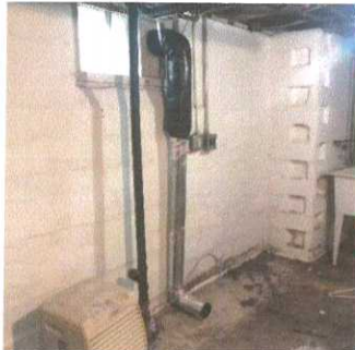
Dryer Vent (6/6) 08/28/2020 12:22 PM
