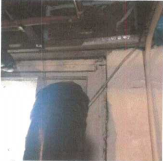
Dryer Vent (5/6) 08/28/2020 12:22 PM
