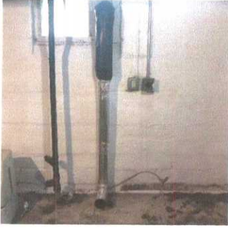
Dryer Vent (1/6) 08/28/2020 12:22 PM
