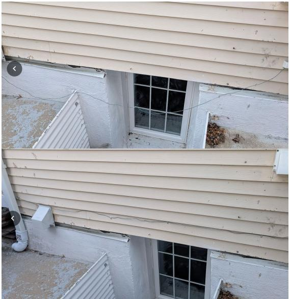
• Remove ground wire in front of Emergency Escape and Rescue Opening on west side of house. \*This outdoor ground wire on the 733 Home is mounted from Xfinity's Network Interface Device (NID) to the electrical meter to hold the fiber connection. This wire has been secured on the home with metal clips and screws and no longer hangs.
