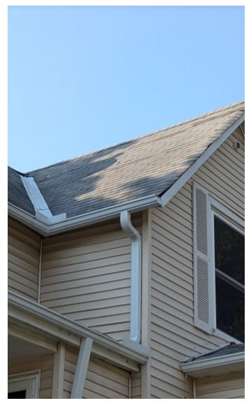
• Two shingles appear to be missing on the roof (NE corner of house – visible from street. Confirm they are not different colored shingles or repair to code.
