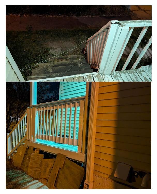
• Front step descending towards the alley from the porch – remove the flight of stairs in its entirety and install a guard rail along the porch OR repair the stairs to code.
