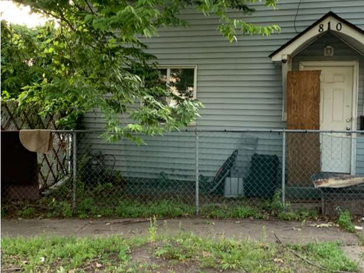
810 Buffalo St.recheck photos 9-10-24
