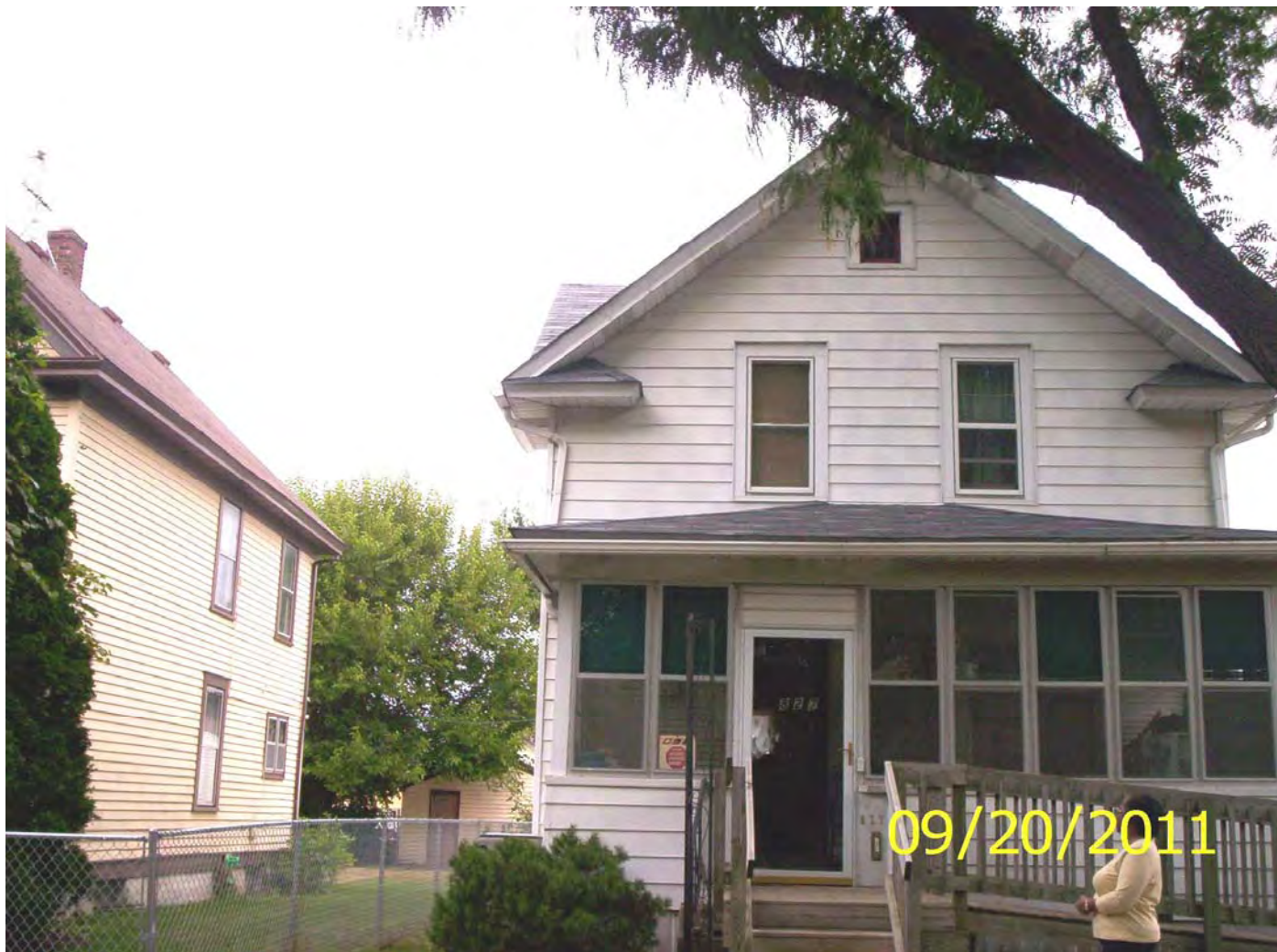
South side of house that was secured
