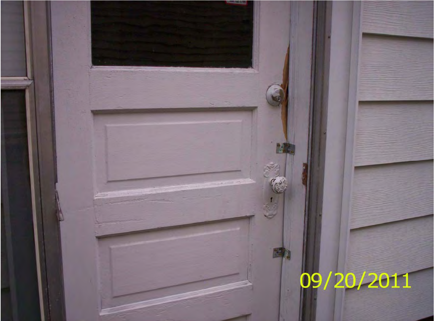
Opening secured – west side door of house
