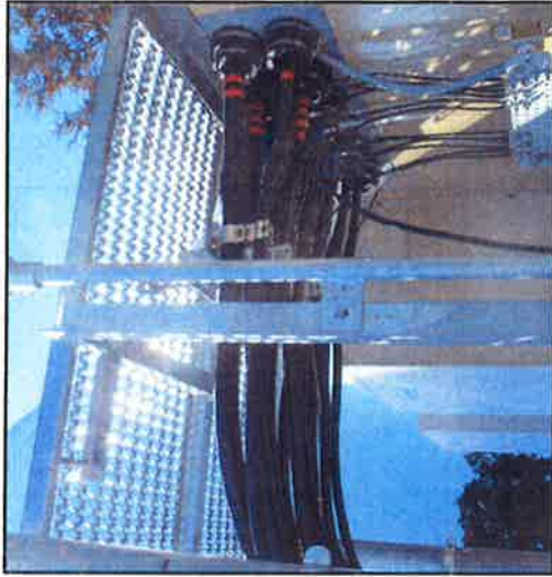
1 CABLE BRIDGE PHOTO SCALE: NONE
