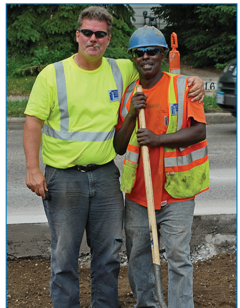
Pete Davis and Wilbert Taylor on a job site in 2008.
