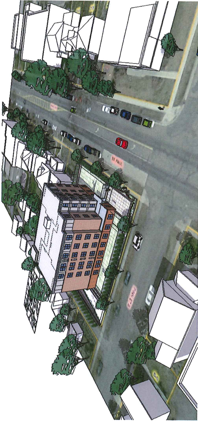
AERIAL VIEW FROM NORTHEAST
