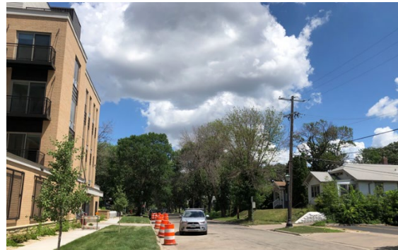
Figure 2: Liffey Apartment Building at Snelling & Carroll Avenue
