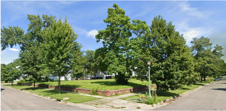
Brownstone retaining wall wrapping the corner
