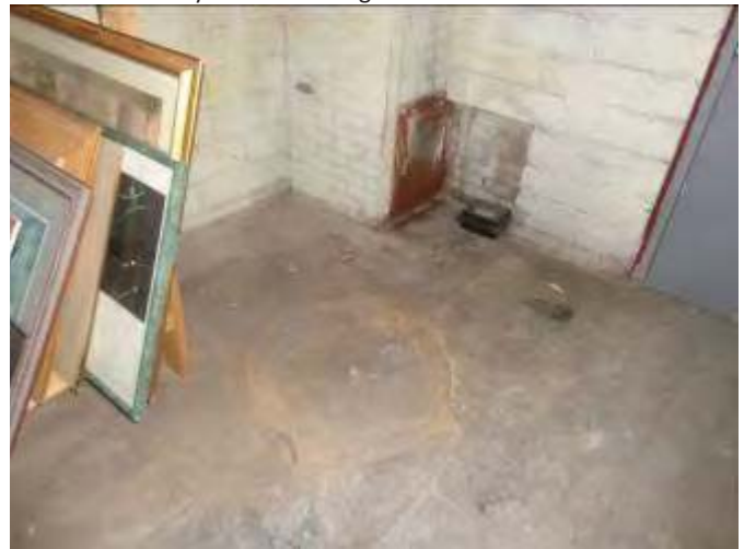
16. Apparent coal shoot/furnace (633 University Ave W)
