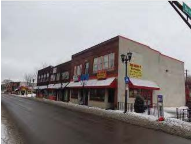
1. Overview of Property, view northwest
