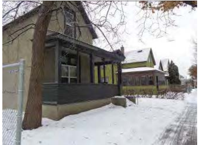
2. North Property boundary and Sherburne residences (628, 632 Sherburne Ave), view west
