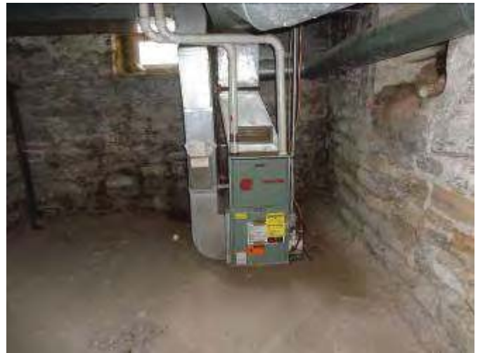
34. Basement and furnace of the residence (628 Sherburne Ave)
