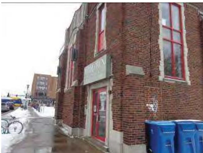
29. Overview of 501 Dale Street North building (Midtown Business Center), view south/southwest
