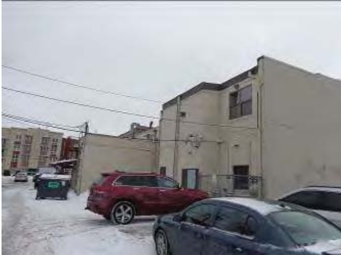
13. Overview of the 625-633 University Ave W buildings, view southeast
