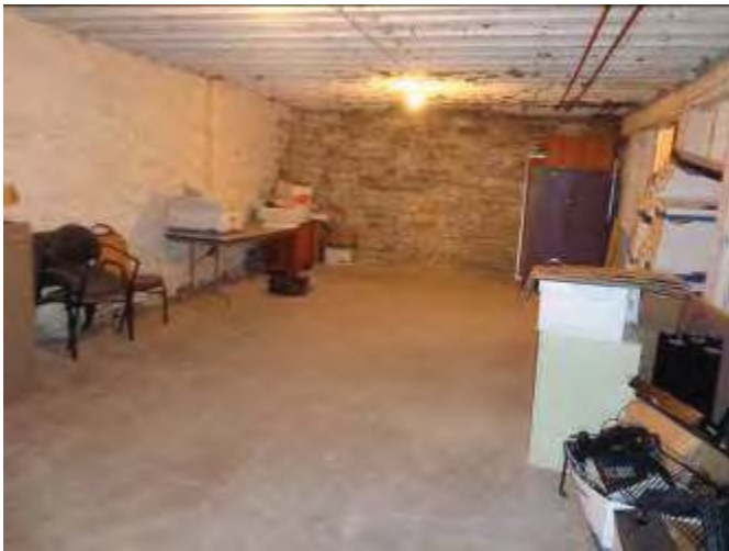
15. Representative basement area (633 University Ave W)
