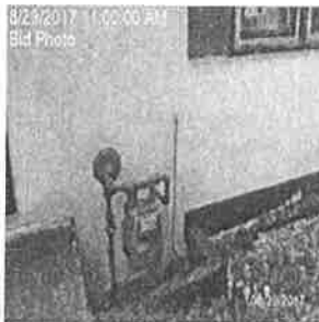
Bid Photo 08/29/2017 HVAC Inspection 2096 Reaney Ave E Saint Paul , MN 55119
