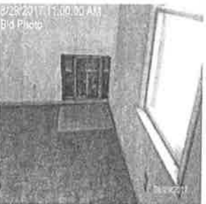
Bid Photo 08/29/2017 Plumbing Inspection 2096 Reaney Ave E Saint Paul , MN 55119
