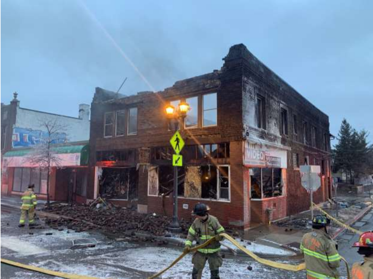
916-918 University Ave W.Fire Photos 1-10-24
