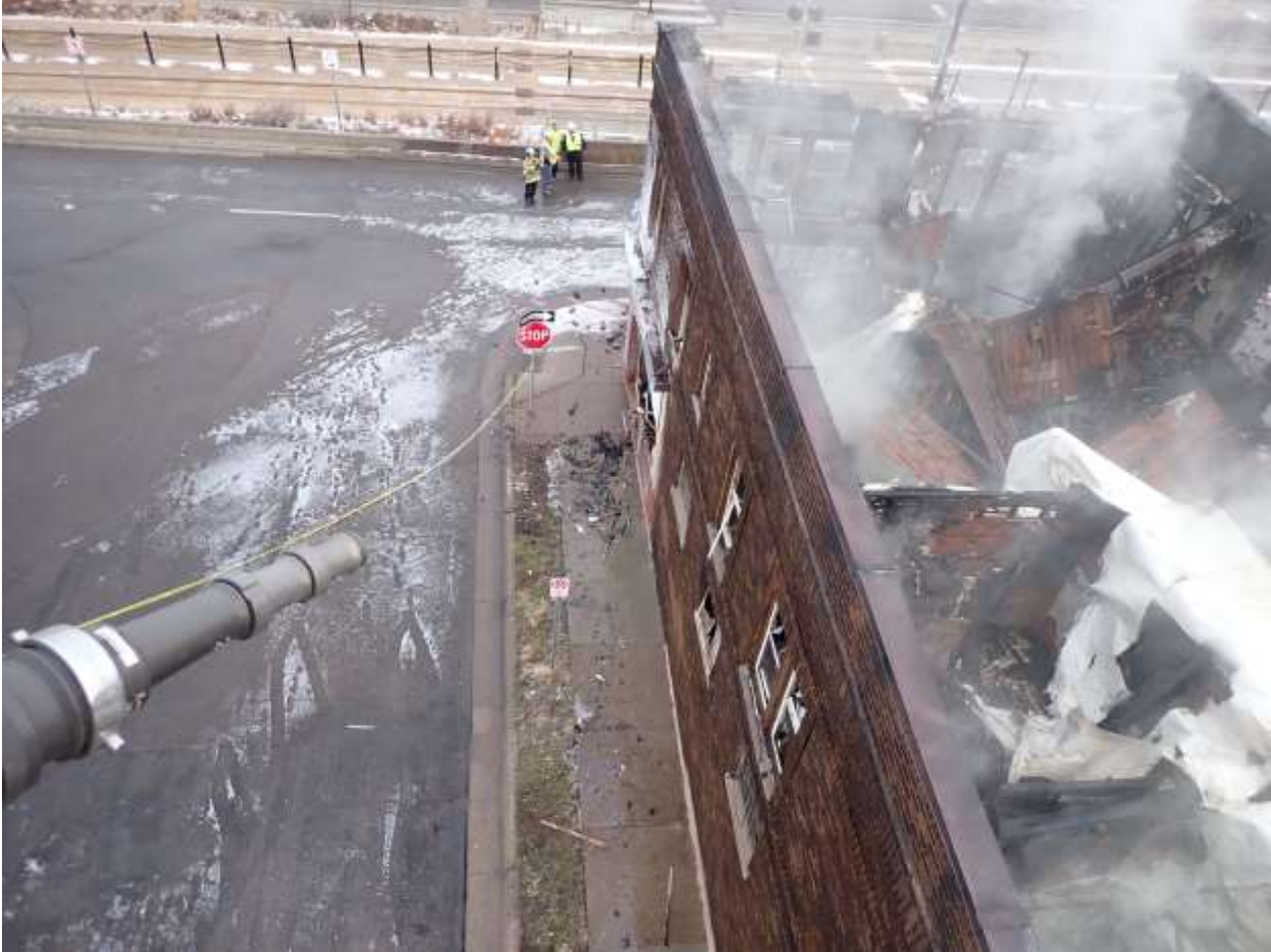
916-918 University Ave W.Fire Photos 1-10-24
