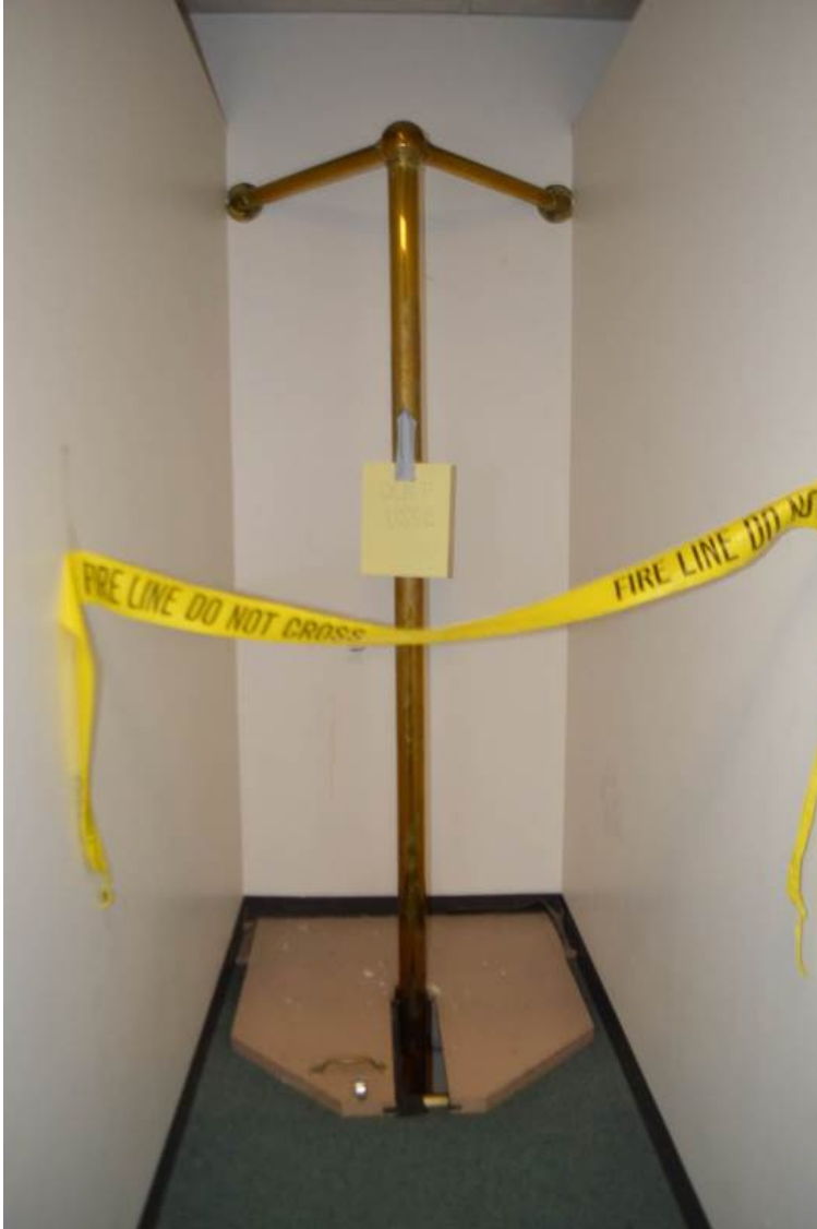
Photograph 15. Fire pole, photograph facing east, taken from upper level.
