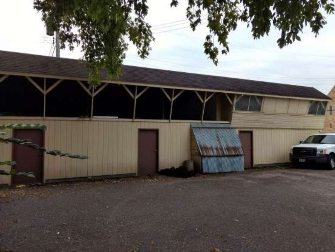
Photograph 7. North façade of shed, camera facing south.
