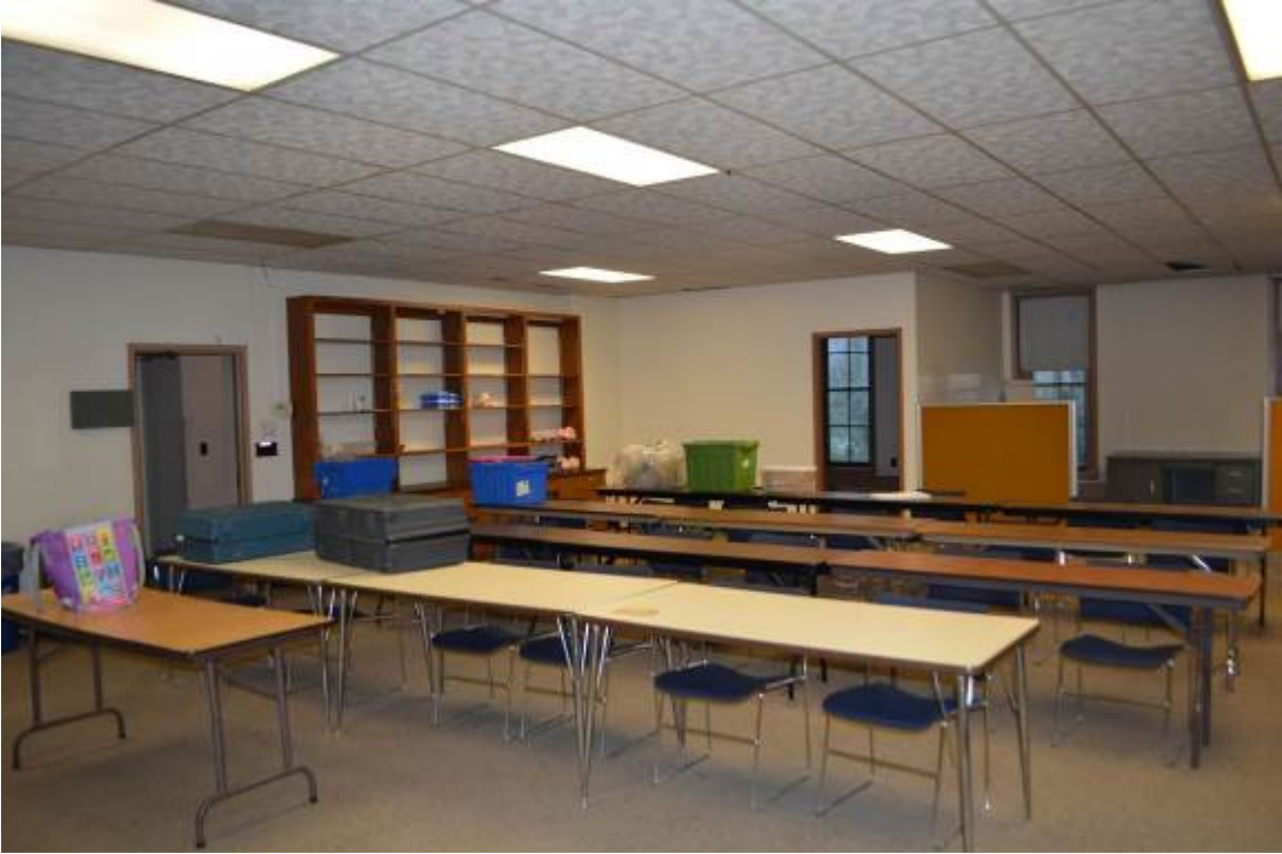
Photograph 14. Classroom on upper level, camera facing northwest.
