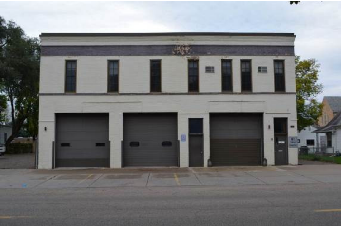
Photograph 1. North façade of Engine House No. 10, taken from Randolph Avenue.
