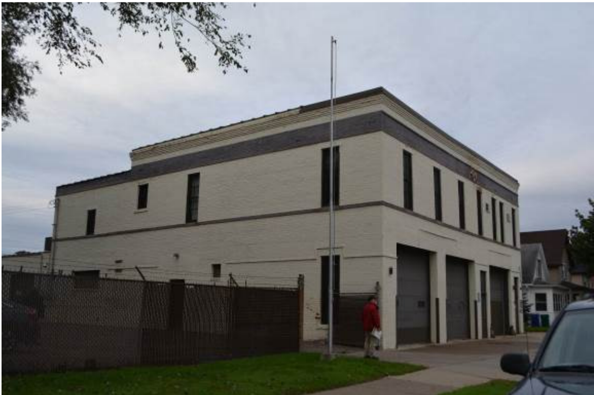
Photograph 3. East façade of Engine House No. 10, taken from Randolph Avenue.
