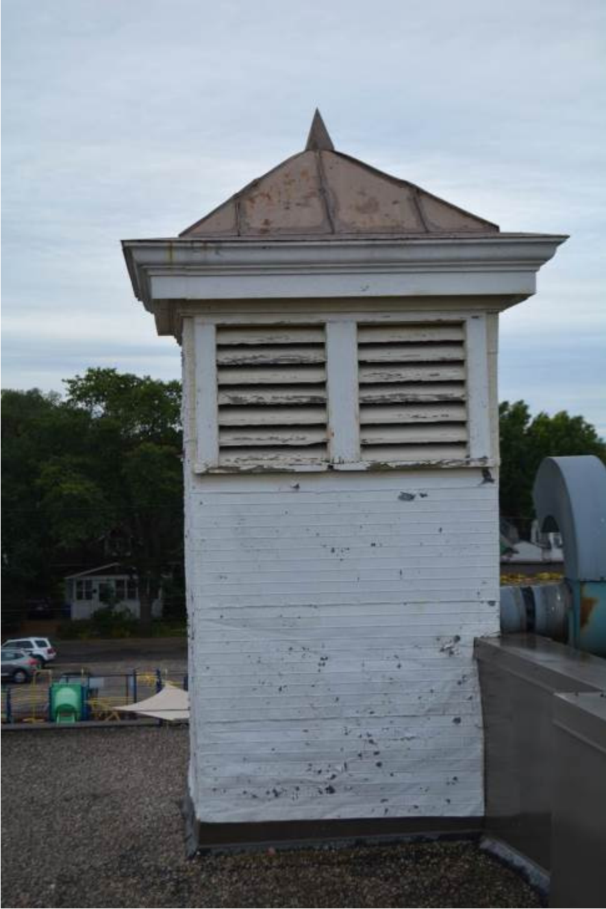
Photograph 6. View of hose tower from roof, camera facing north.
