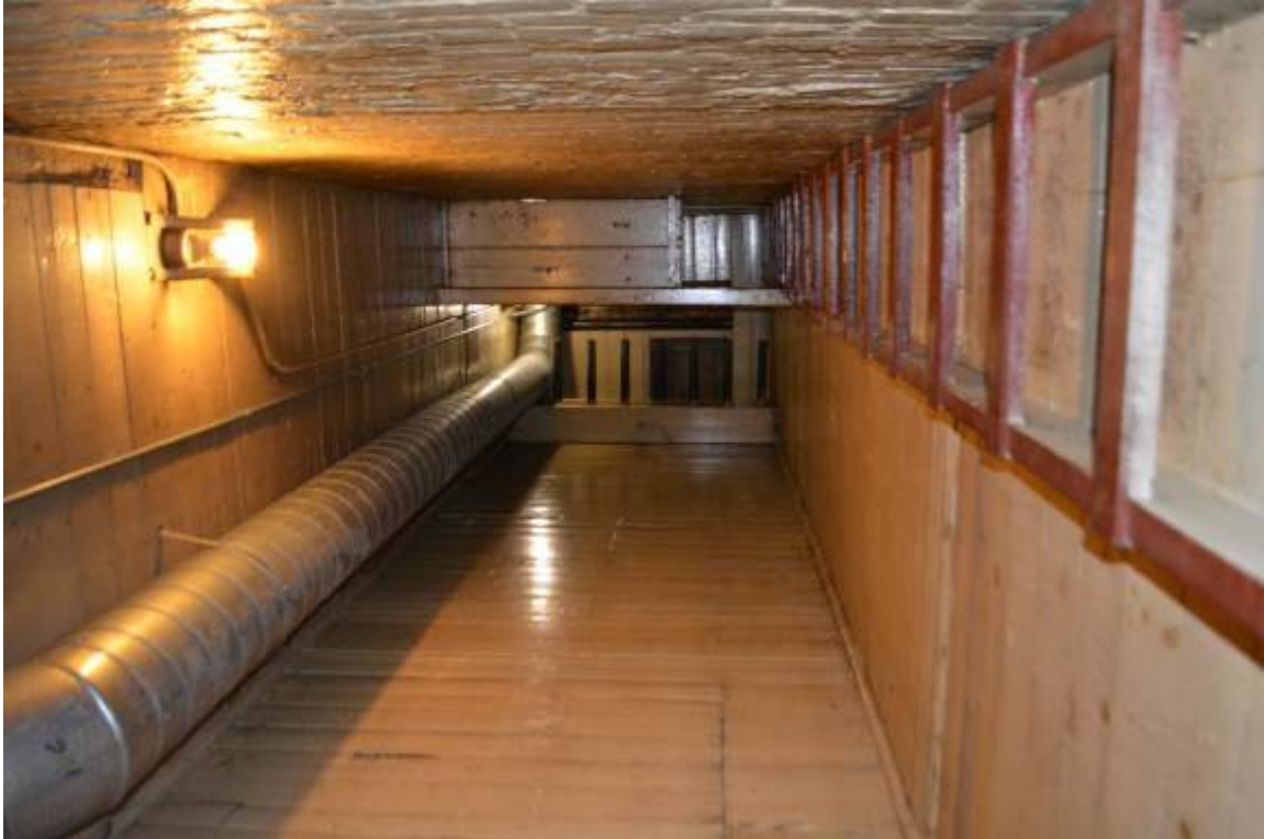
Photograph 12. Interior of hose tower, looking up from main level.
