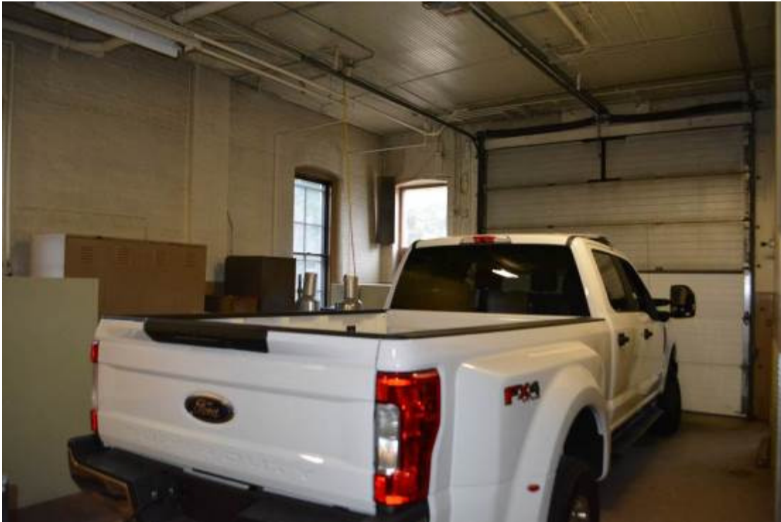
Photograph 9. Interior of 1911 apparatus bay, camera facing northwest.
