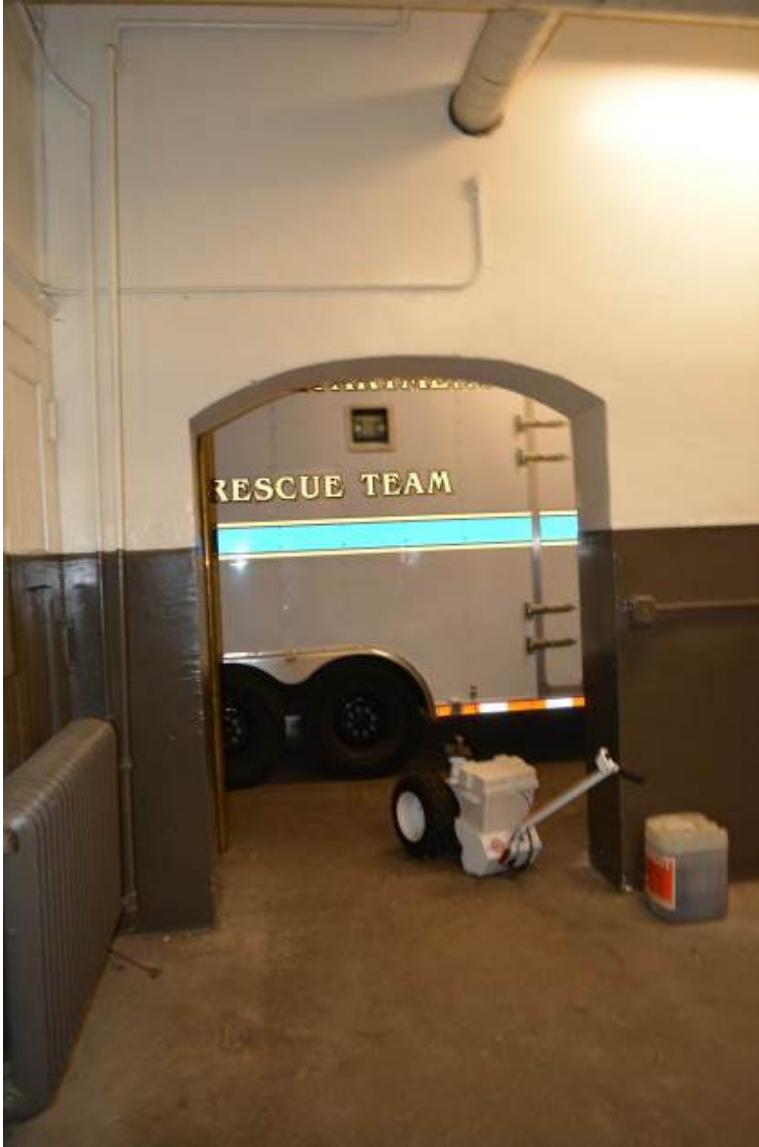
Photograph 10. Brick arch passage between 1885 building and 1911 addition, camera facing west. Photograph taken from 1885 apparatus bay.
