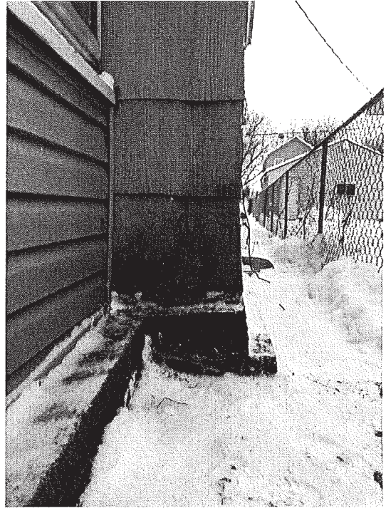
Photo 2 – Poured Concrete Ledge at Perimeter
