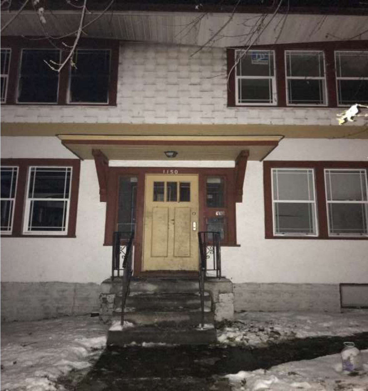
1150 Central Ave W.Photos
