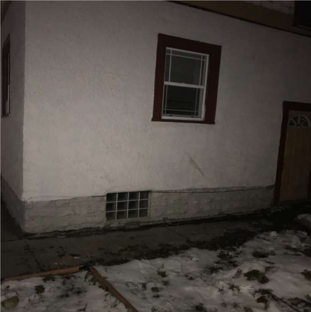
1150 Central Ave W.Photos
