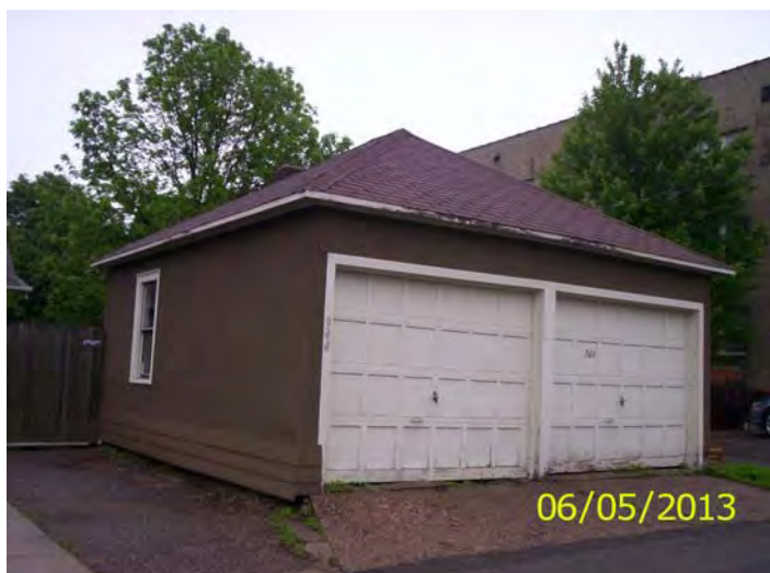
East side garage
