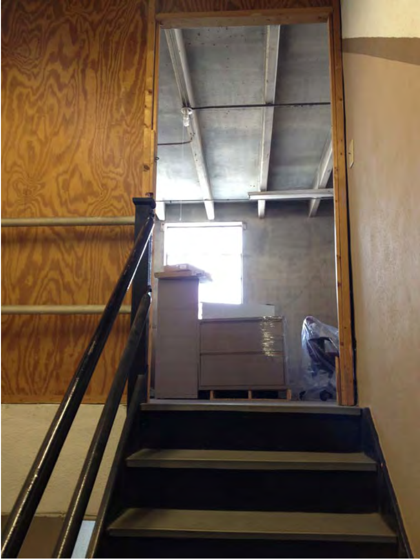
Opening at 3 rd floor taken from stair side.
