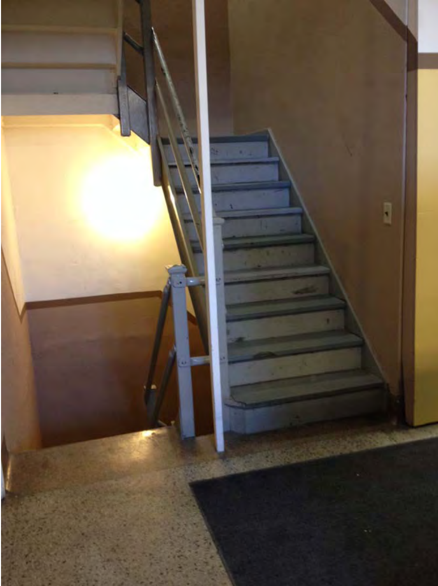
Opening at 1 st floor. No landing or lobby area. Next picture is an enlargement of the bottom right of this picture.
