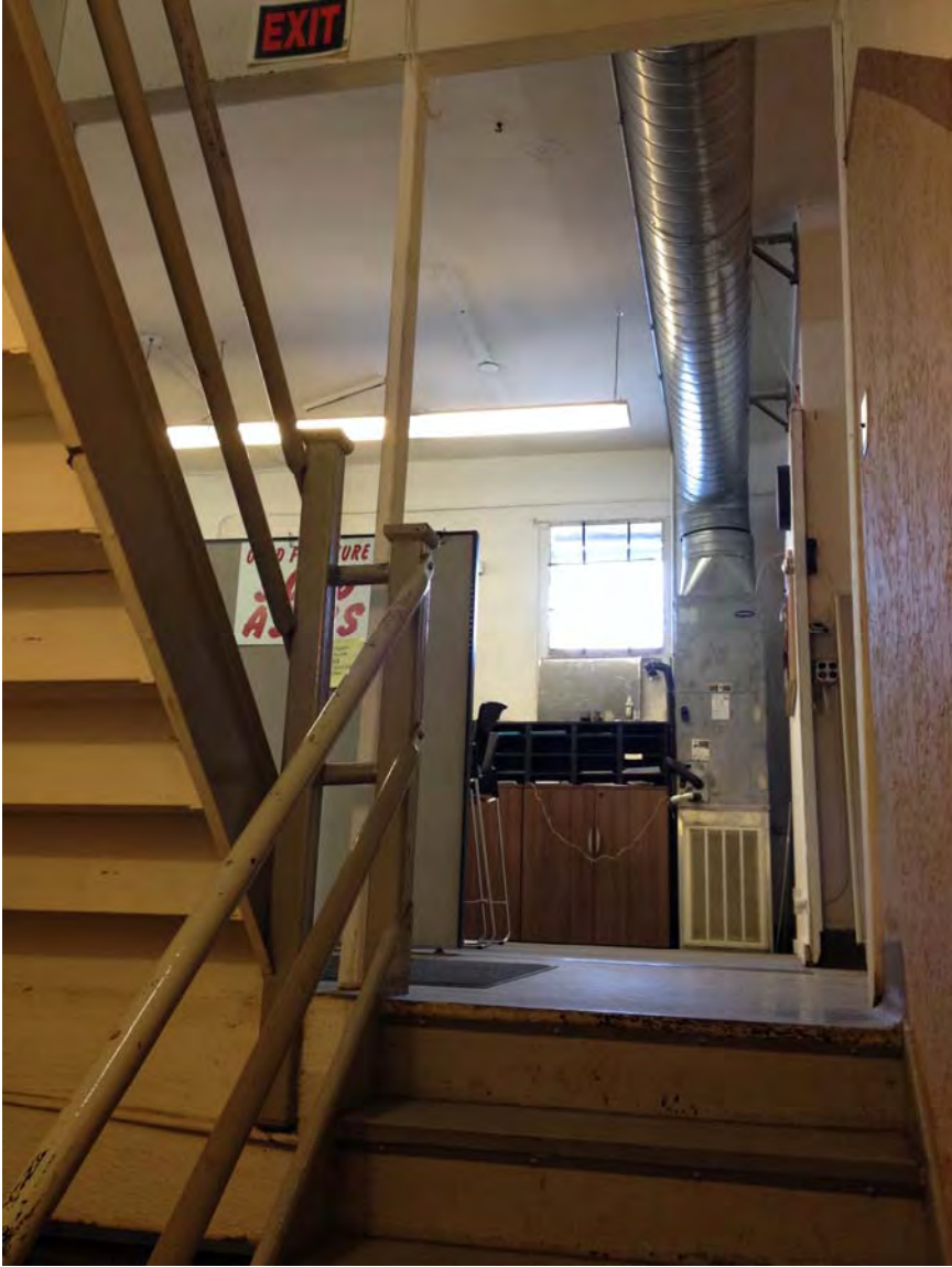
1 st floor opening from the stair side.
