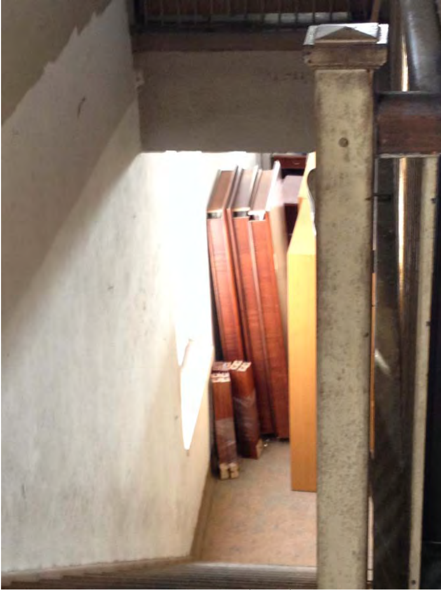
A second open stair that goes from 3 rd to 2 nd floor.
