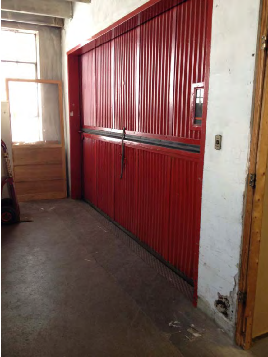
Freight elevator at 3 rd floor
