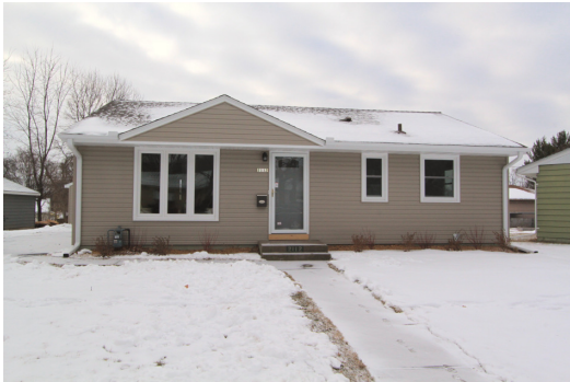
2112 Ivy Avenue E. Attachment C – Photos
