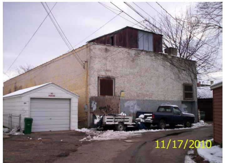
North side and east sides
