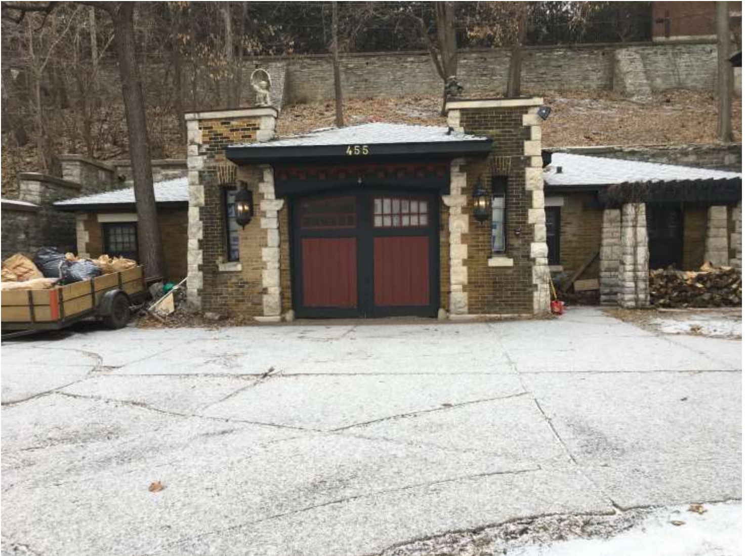
Front of the carriage house again.
