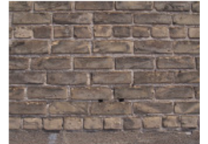
3 - SOUTH BRICK CLOSE UP
