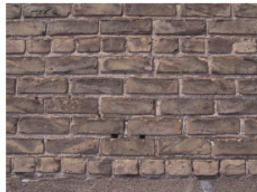
3 - South & West Brick
