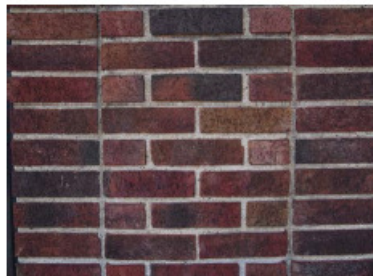
1 - North Brick Existing Building Material Palette
