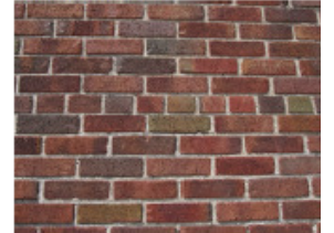
2 - EAST BRICK CLOSE UP
