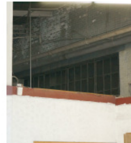
4 INTERIOR VIEW, INTERIOR COVERED UP BELOW 8'-0" A.F.F. W/ MAN DOOR
