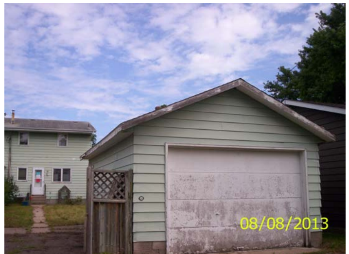
Garage, south side, posting
