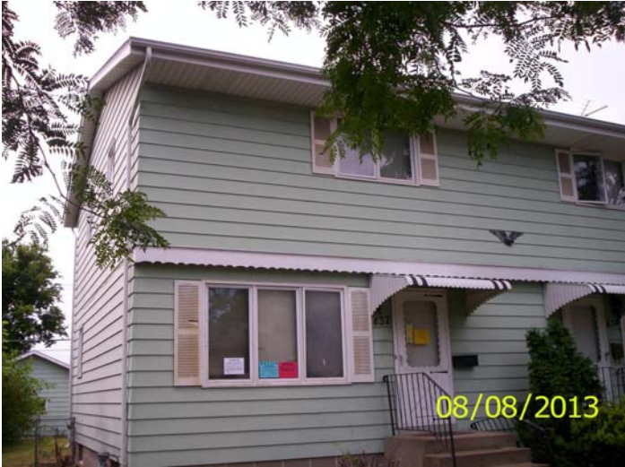
North and east sides, posting
