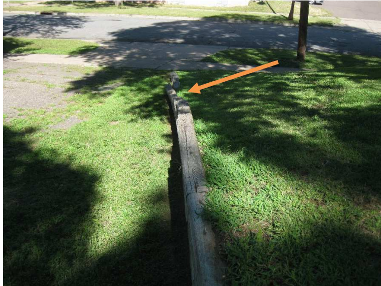
Picture 9 – Timber Retaining Wall
