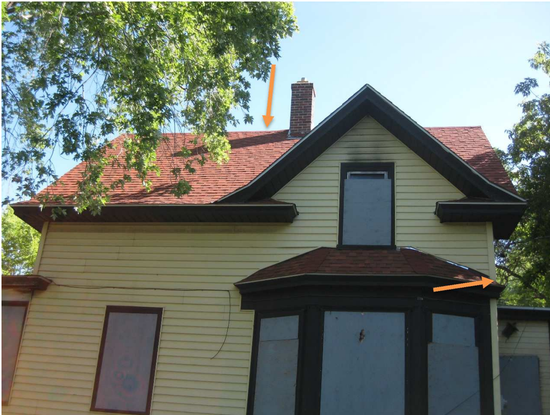
Picture 13 – House Roof and Exterior Wall
