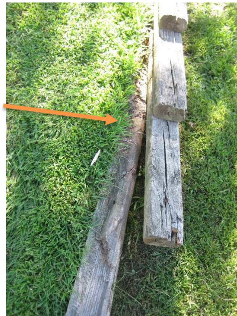
Picture 10 – End of Timber Retaining Wall
