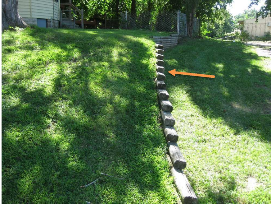
Picture 11 – Timber Retaining Wall
