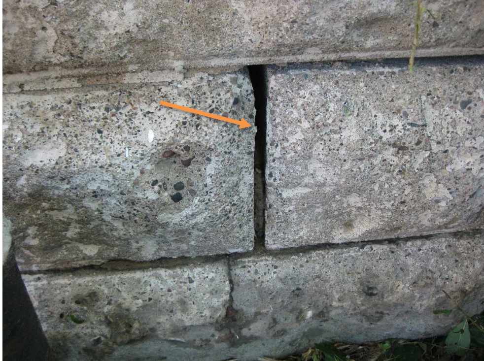
Picture 7 – Exterior Foundation Walls
