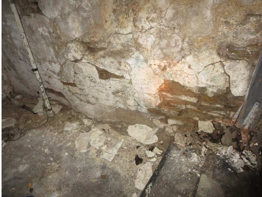
Picture 5 – Interior Foundation Wall
