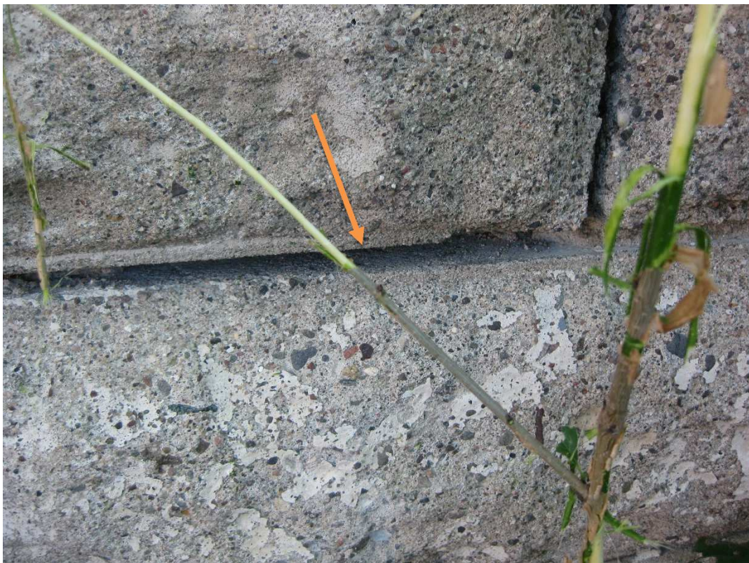
Picture 8 – Exterior Foundation Walls
