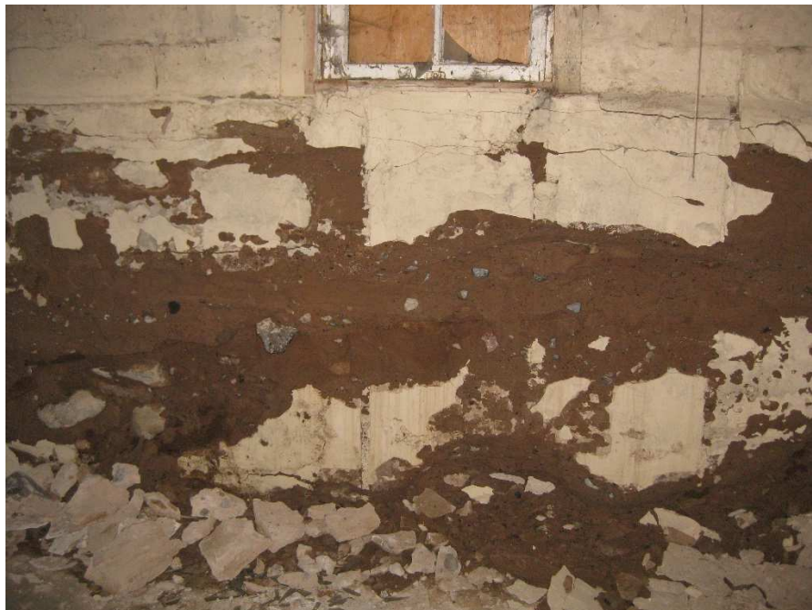
Picture 6 – Interior Foundation Wall
