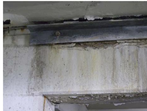
Close up of concrete under angle
