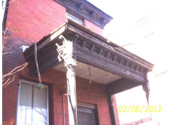
Roof over the rear deck
