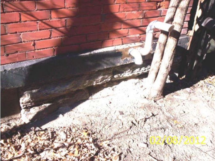
Deteriorated foundation
