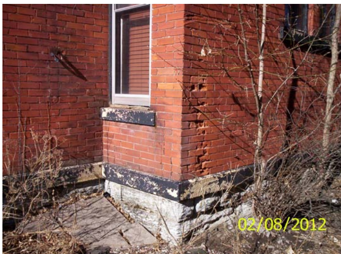
Deteriorated masonry
