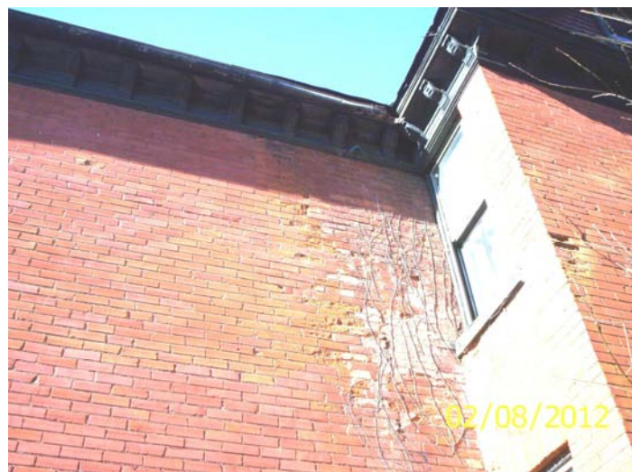
Deteriorated masonry
